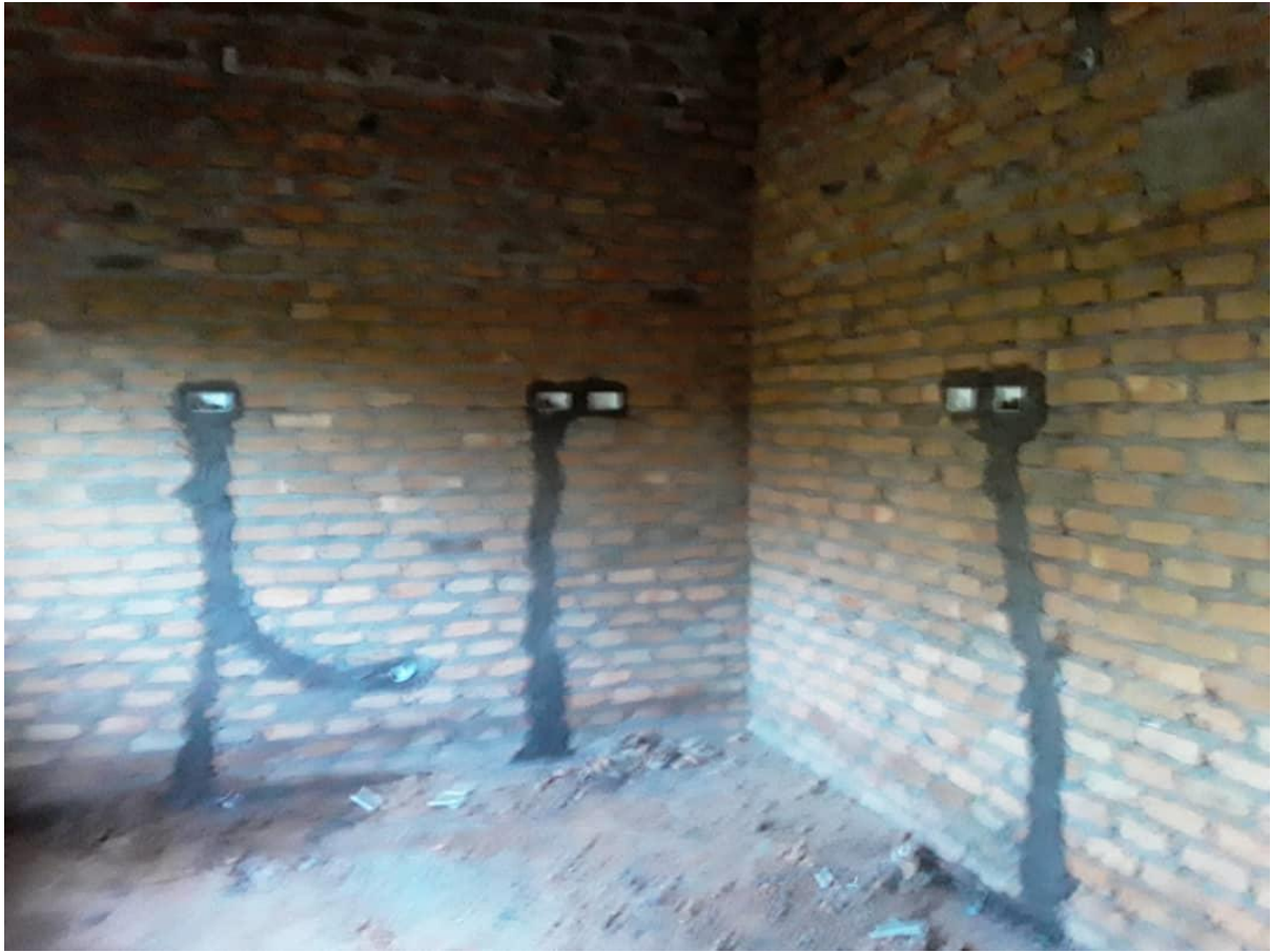
Some electrical components fixed to the wall before plastering is done
