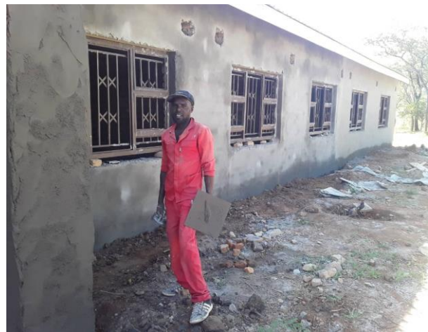
Plastering of the facility taking place. Window frames already fixed to it
