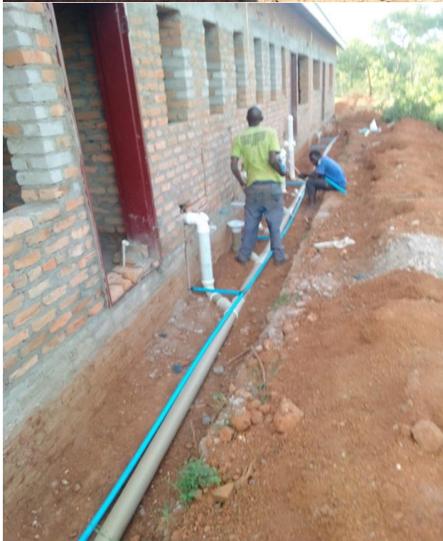
Plumping work being carried out before plastering was done
