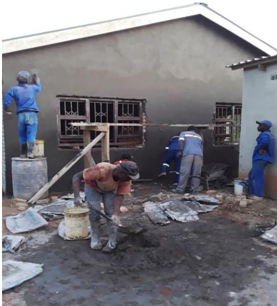
Plastering of the facility taking place. Window frames already fixed to it
